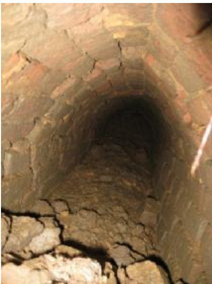
The brick culvert in the eastern edge of Trench P.
