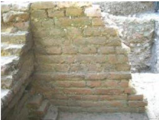
*Cleaned-up walls showing the variations in brick sizes and bonding.*
