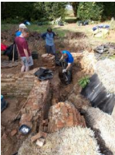
Carefully excavating the surface of the brick drain under the walkway next to the garden wall. Also visible are several of the related support pillars and a vertical brick drain in the background, with a substantial brick structure going off to the left.
