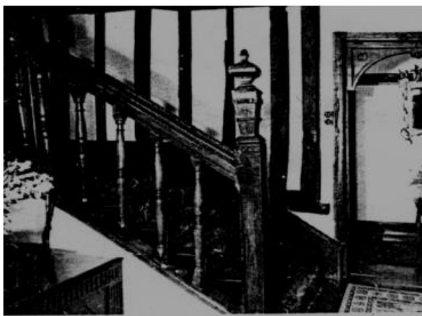
The staircase at Priors. c1600
